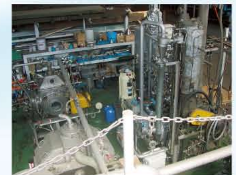
Test site and various test machines
